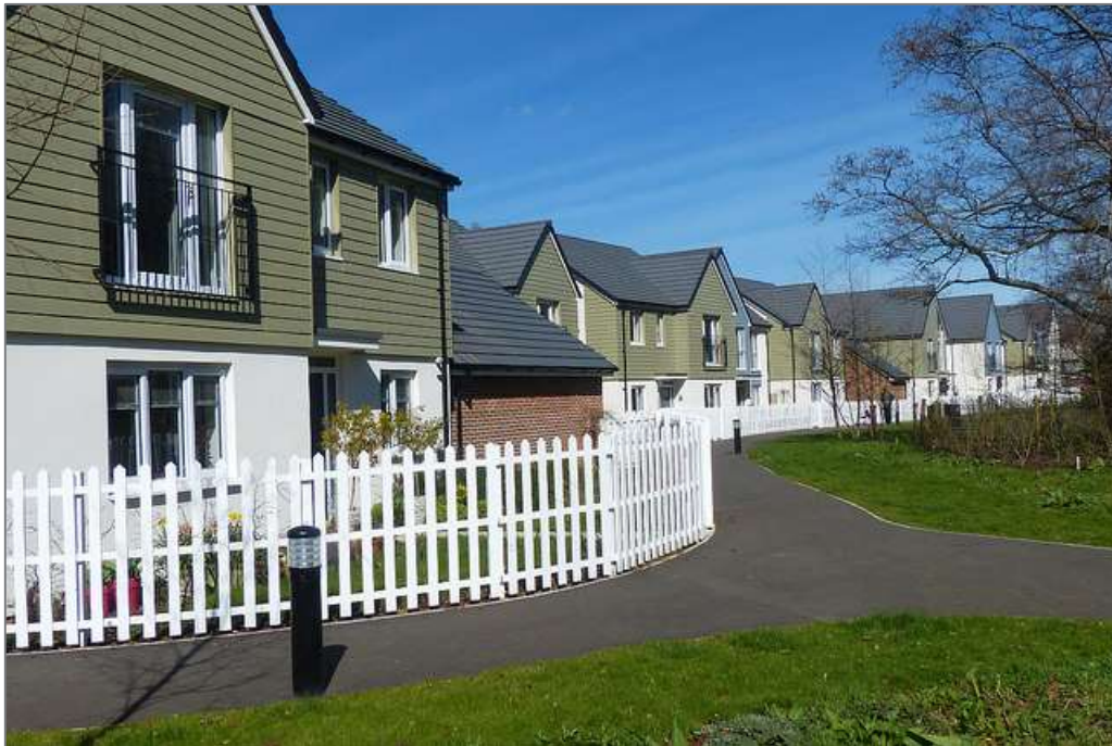
FIGURE 19: NEW HOUSES AT GLAN LLYN H1(47)
