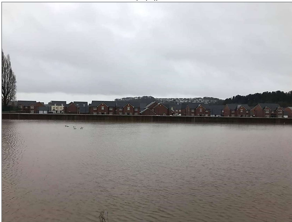
FIGURE 14: FLOOD DEFENCES AT JUBILEE PARK (H1(54)) FOLLOWING STORM DENNIS IN FEBRUARY 2020
